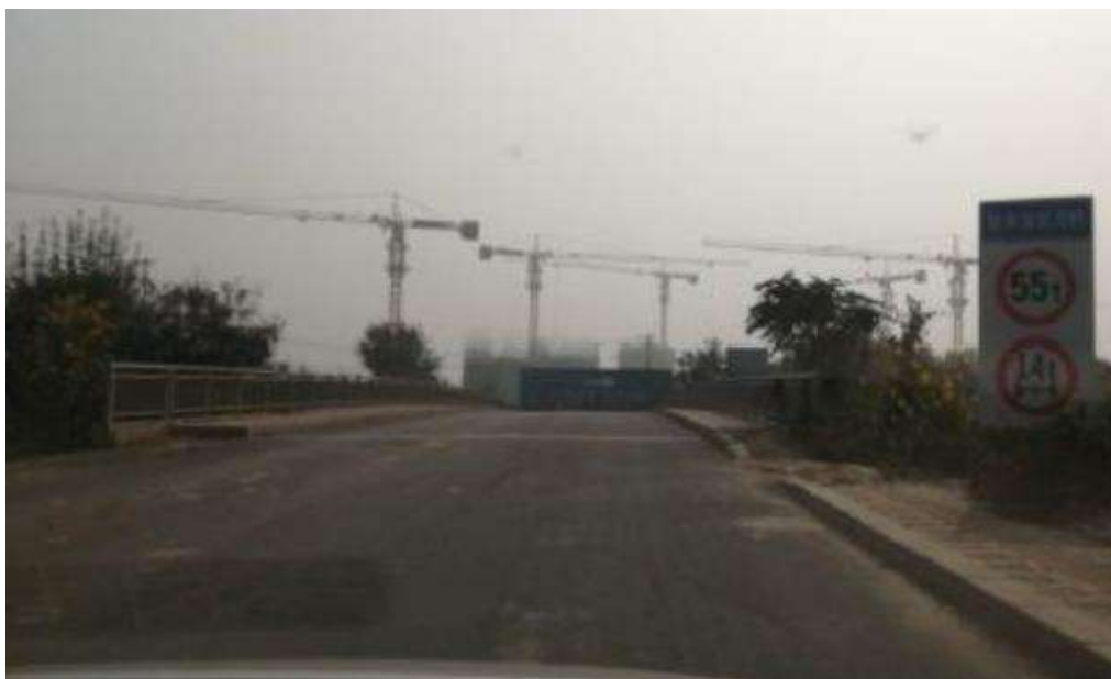
图 2-1-2 现状白万公路跨洪泥河桥
